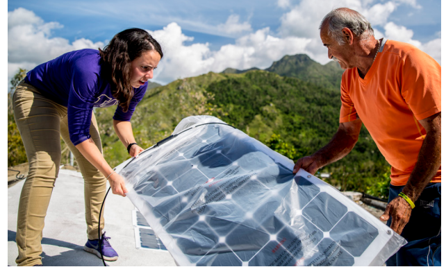
CEI Graduate Fellow Mareldi Ahumada-Paras (left) and a homeowner install solar panels in Jayuya, Puerto Rico after Hurricane Maria.
